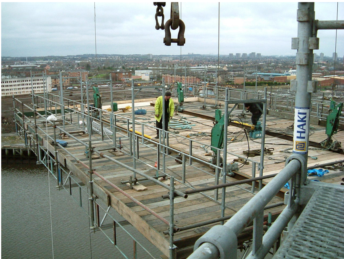
Early stage work building the access platform high above the water
