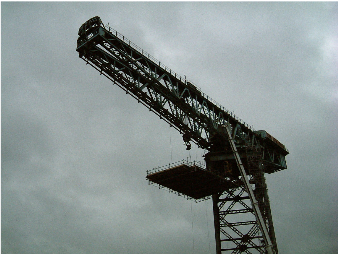
Working platform being lifted into position
